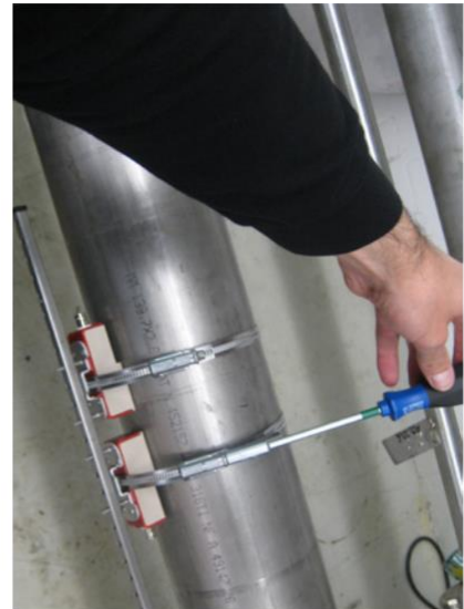
Transducer installation: quick and easy
